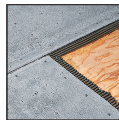
Stagger surface and panel joints
