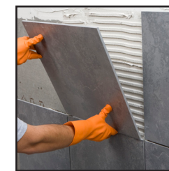
Press tiles into place
