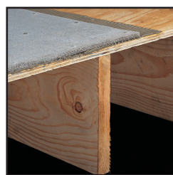
5/8" subfloor with 16" on center framing
